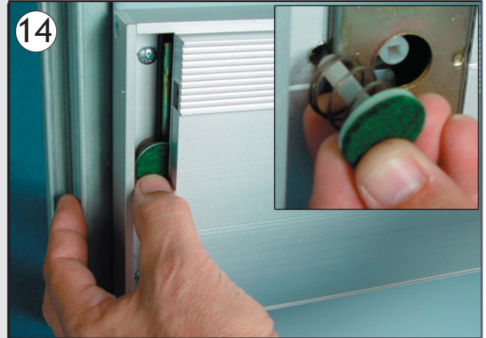
Insert the panic button as shown in inset picture. Slide the bar over.
