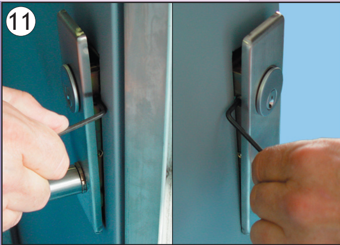
Tighten the allen set screws on both sides of the lock.
